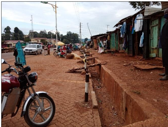
Constructed storm water drainage channel
