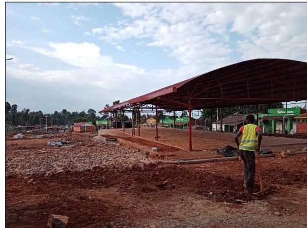
Miruka Market under construction
