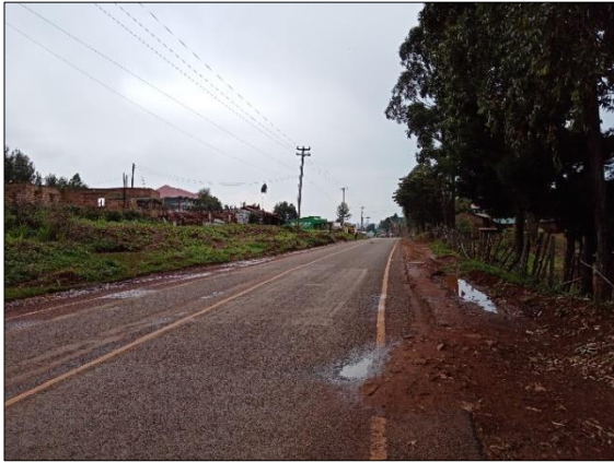
Bitumen road in Nyamira Municipality (Konate –Senta Road (B5))
