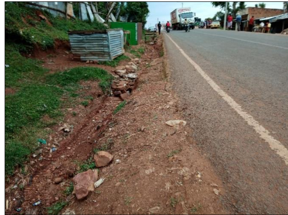
Dug storm water drainage channel
