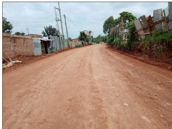
Well maintained earth road
