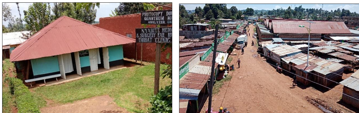
Plate 24: Common roofing material within the municipality
