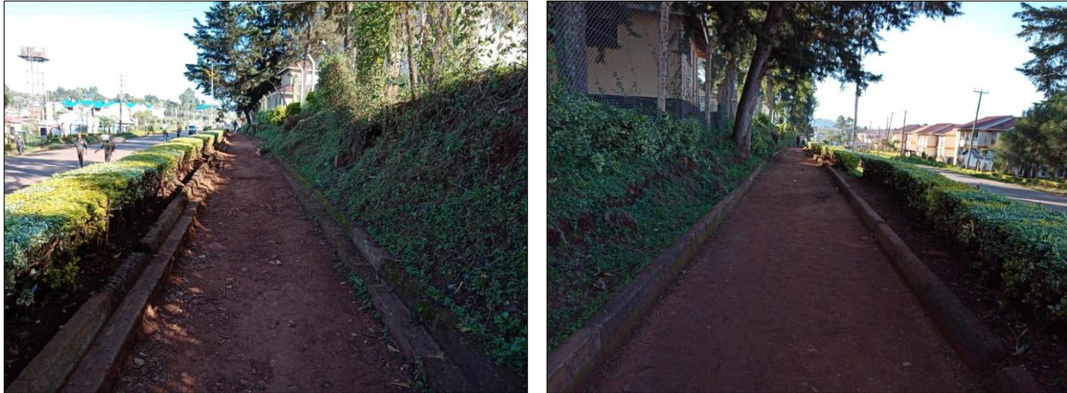
Plate 17: Pedestrian walkway along Konate-Senta road (B5)
