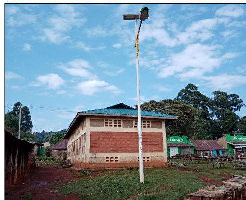
Solar Powered Street light at Nyamaiya
